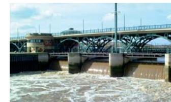
The main priority of the barrage is to control the flow of the river, protect the surrounding areas from flooding, and prevent any other effects of tidal change.
