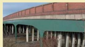
Built as part of the northern approach road to Newport Bridge, this was the first all-welded portal frame bridge in the world. It has a central span of 19.6m with 14.6m and
