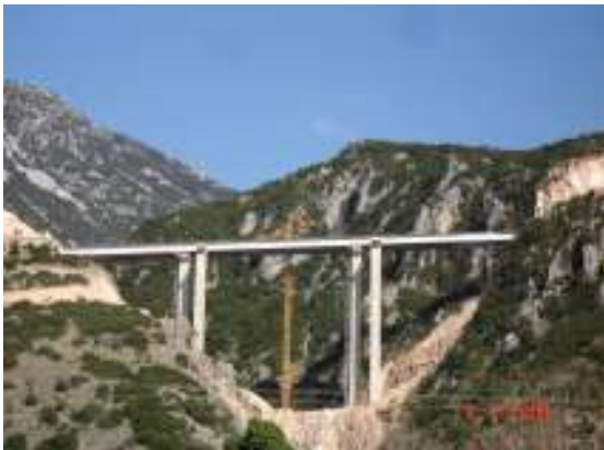
View of the bridge
