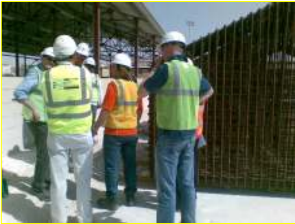
Pumping Station Site Visit
