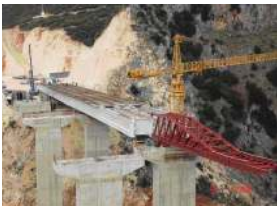
View of the steel nose of the steel beams
