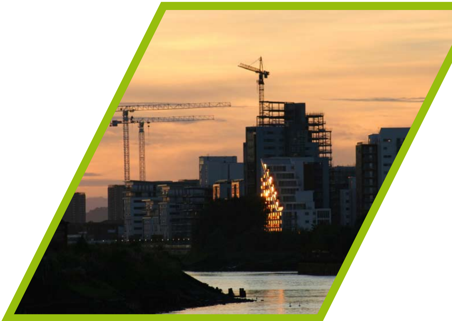
Figure 5. Aerial view of the Glasgow Harbour regeneration, where Demolition Protocol approaches have led to hundreds of thousands of tonnes of material remaining on-site and being recycled.
