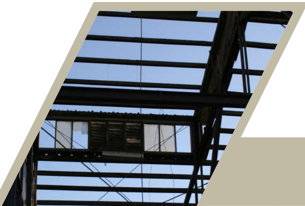
Figure 8. A steel-framed structure being deconstructed
