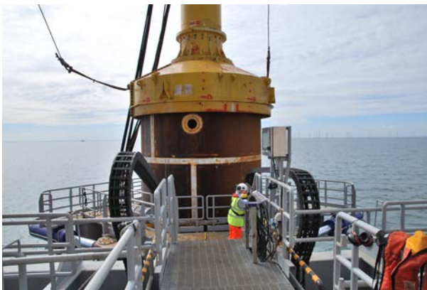
Hammer on Pile Follower, Pile Follower held by Pile Gripper
