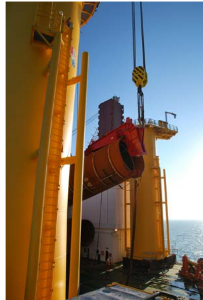
Upending Monopile from cradles on deck of jackup. Transition Pieces visible in foreground and background
