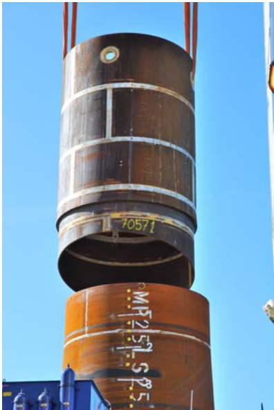
Placing Pile Follower on Monopile (Monopile is resting on seabed and is held by Pile Gripper)
