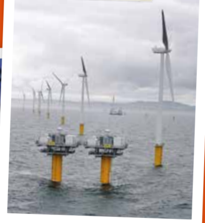
OFFSHORE WIND FARM
