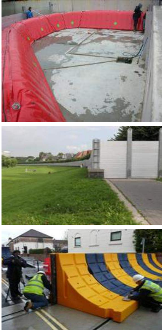
Figure 3 Temporary and demountable perimeter flood barriers
