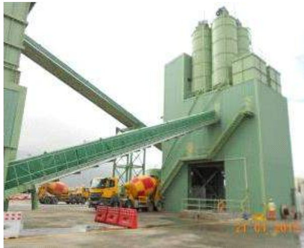
Figure 7 Concrete batching plant in MFC construction site
