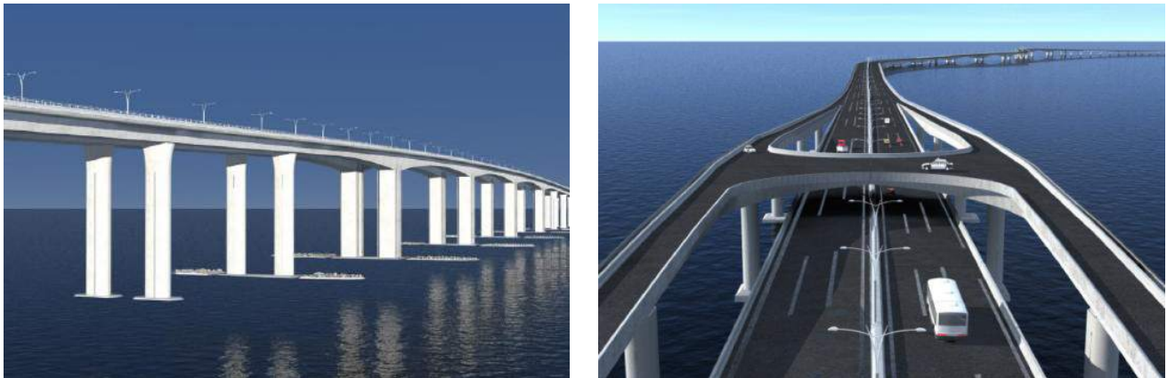
a. Viaducts in Western Waters
