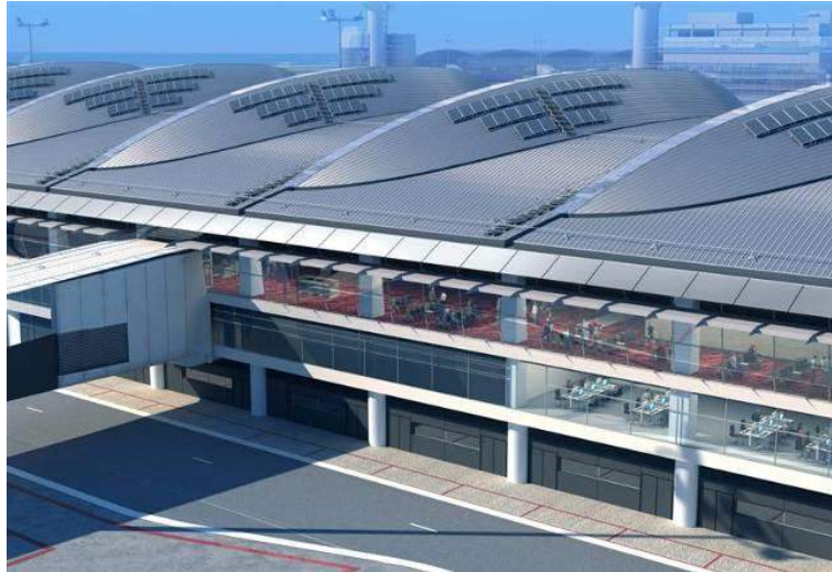
Figure 11 PV panels at MFC
