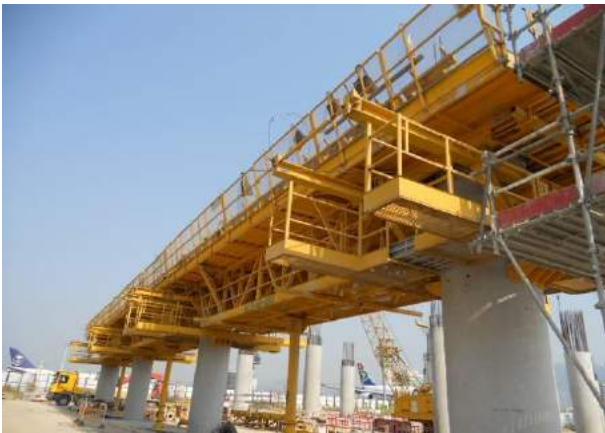
Figure 4 Beam shutter used in MFC
