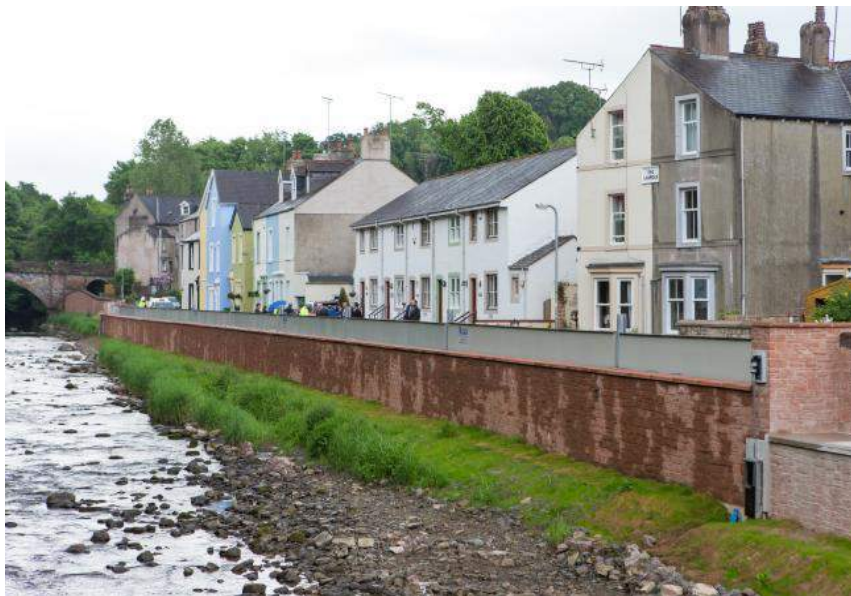
Figure 5 Flood defence barrier
