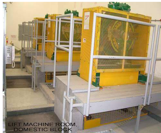
Figure 6 Gearless permanent magnet synchronous lift motor
