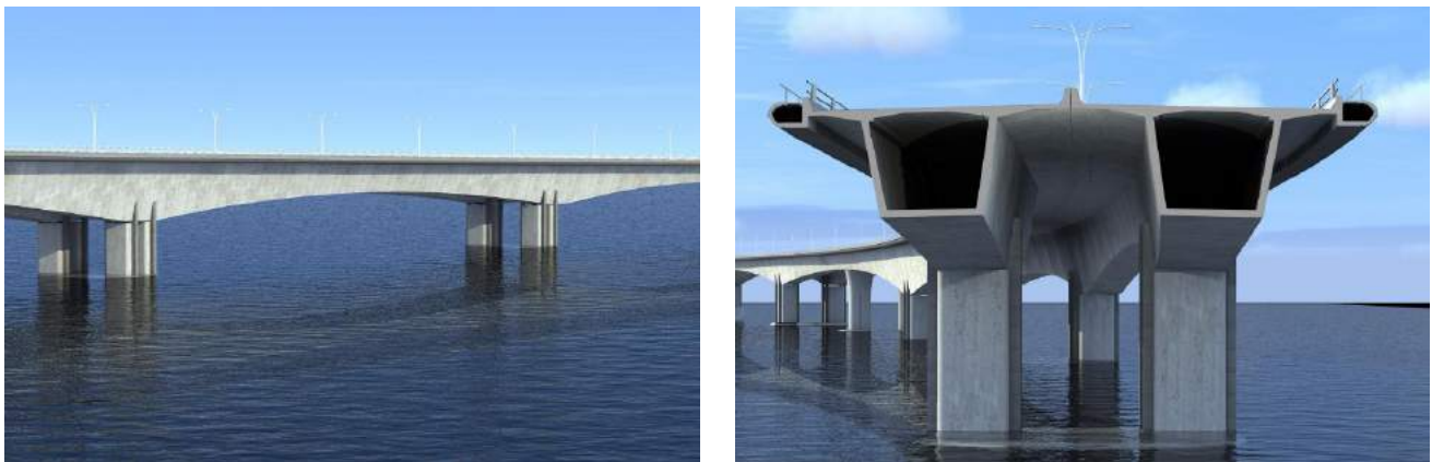
b. Viaducts in airport channel &amp; headland
