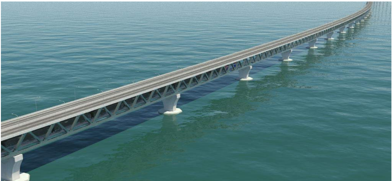
Figure 8 Padma Bridge – a two-level rail-road bridge
