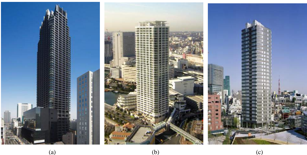
Figure 18 (a) The Glorio-tower Roppongi, (b) the Nabule-Yokohma tower and residence, and (c) the Kitahama Tower in Osaka are recent tall buildings using ECC coupling beams for structural resiliency (Kanda et al., 2011 and Yamamoto, 2008)
