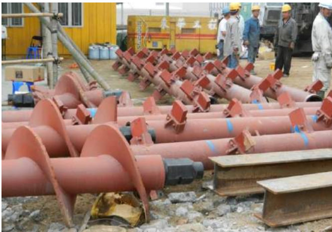
Figure 2 Auger and mixer used for pile installation
