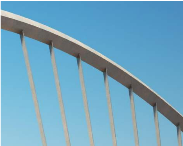
Figure 2 Hook-shaped steel plated hangers
