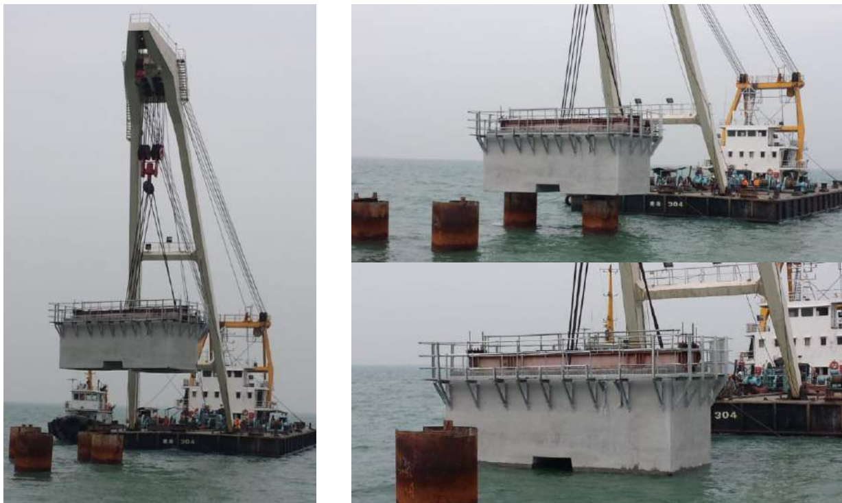
Figure 11 Installation of precast concrete shell for pile cap construction
