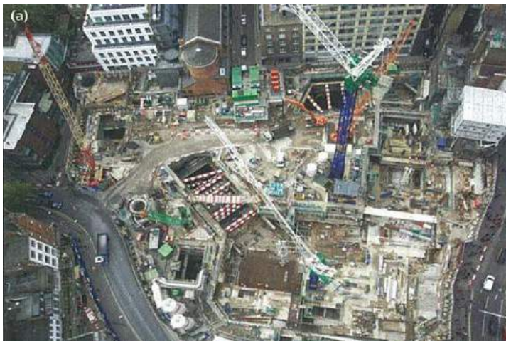
Figure 22 Site photograph of the works (11/12).
