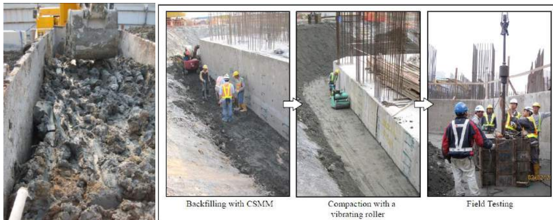
Figure 11 Mixing, backfilling, compacting and field testing of cement stabilized marine mud
