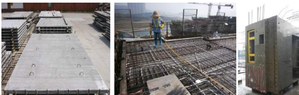
Figure 12 Semi-precast slabs and volumetric precast bathroom in public housing
