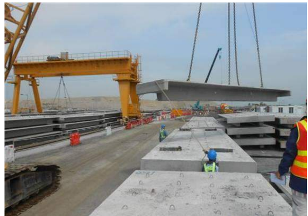
Figure 5 Precast structural floors
