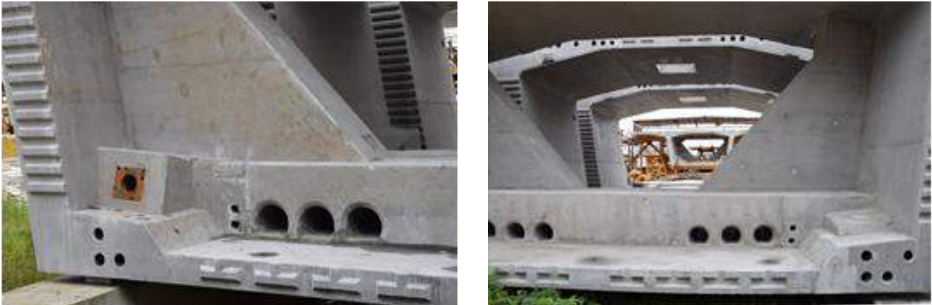
Figure 5 Prestressing ducts for mixed scheme
