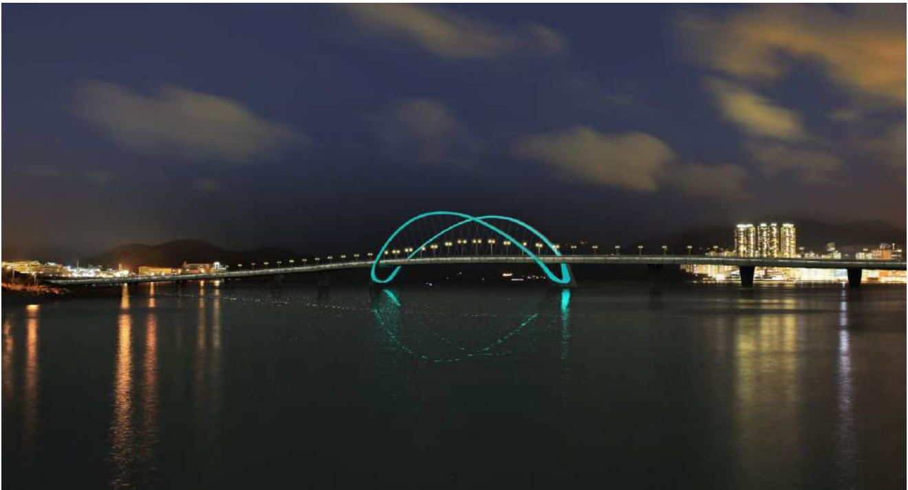
Figure 9 Cross Bay Link Bridge
