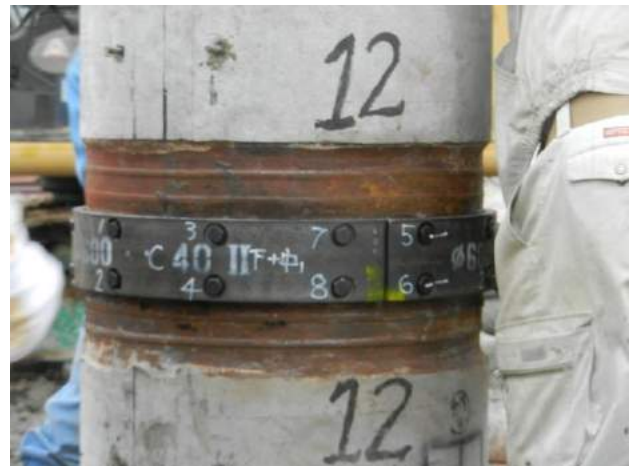
Figure 3 Mechanical splicing of PHC piles
