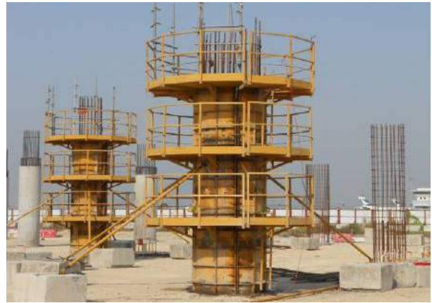
Figure 3 Steel column shutter used in MFC
