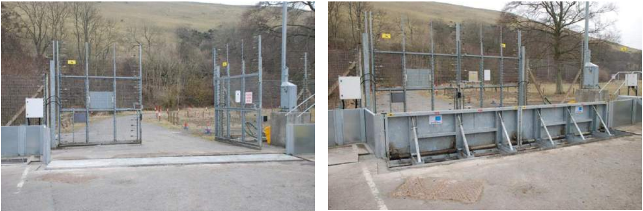
Figure 4 Spring Dam prior to and after deployment: courtesy of TiltDam
