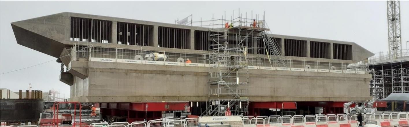
The main cooling water supply for the Hinkley Point C nuclear power station will be fed from four intake heads which will be located on the seabed. Despite the challenges of the global pandemic, the project team were able to complete the construction of the heads at Avonmouth and ensure that the next phase, the transportation of the heads out into the Bristol Channel, remained on schedule.
