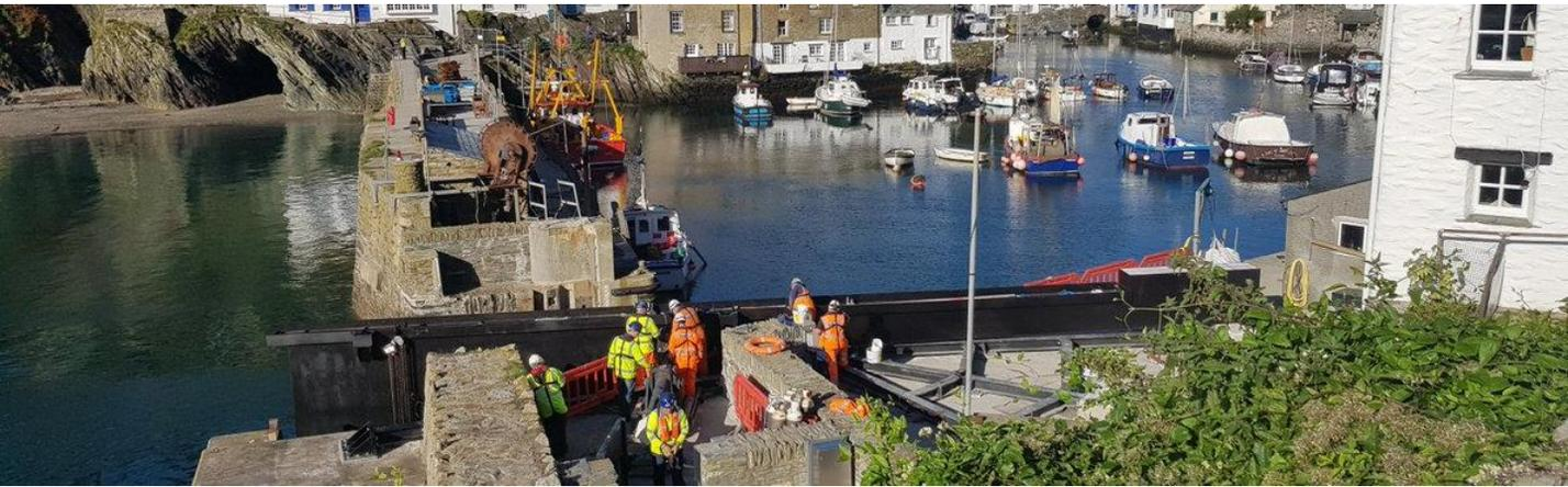
The village of Polperro is a small fishing community with many listed buildings and high tourism appeal. The harbour gate was installed in 1978 and refurbished in 2008 to provide greater flood defence capability. But storms in 2014 damaged the foundations of the gate, requiring a reactive repair. The multidisciplinary partnership project worked to protect people and property from tidal flooding and coastal erosion.
