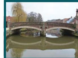
At its northern end is Fye Bridge (7). The present wide two-span bridge constructed of reinforced concrete, masonry and brick replaced an earlier narrower bridge in 1931. There has been a bridge on this site from Anglo Saxon times with the earliest bridges probably being made of timber.
