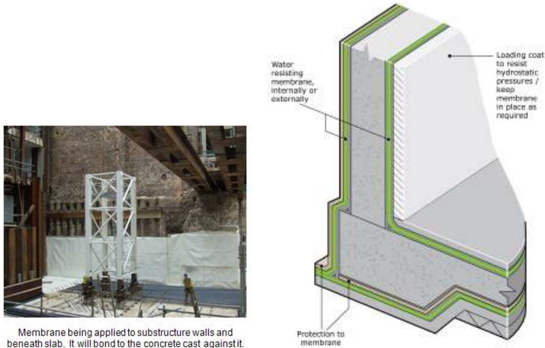
Membrane being applied to substructure walls and beneath slab. It will bond to the concrete cast against it.
