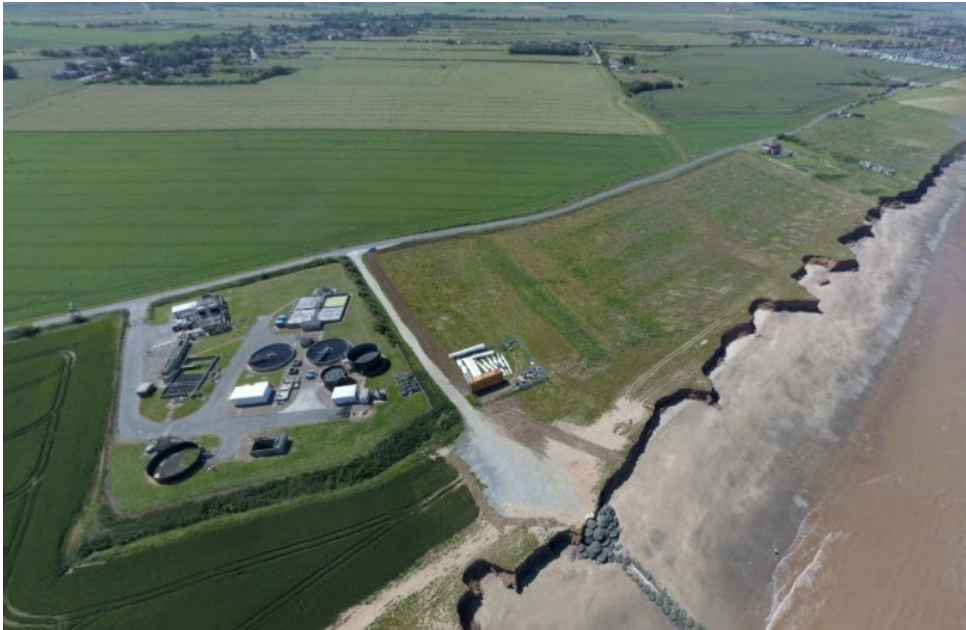
Figure 1 Google image showing the existing STW and cliff erosion
