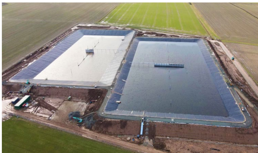
Figure 3: Aerial view of the works nearing completion.
