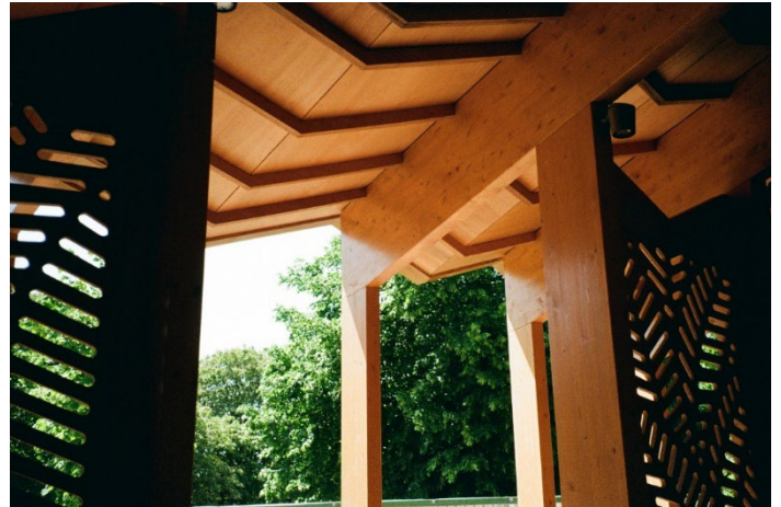
Pavilion entrance showcasing refined detailing and discretely concealed timber connection interfaces throughout
