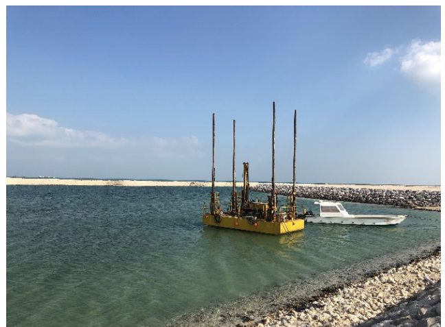
Marine ground investigation at Qetaifan Island, Qatar
