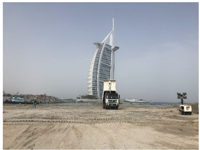
Construction of Marsa Al Arab looking over to the Burj Al Arab, UAE
