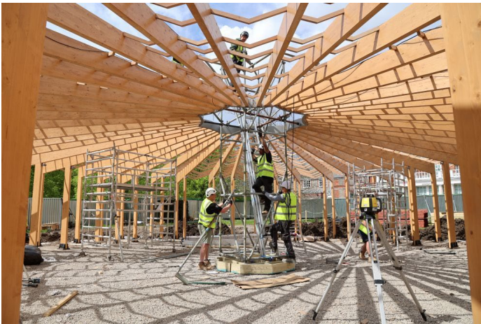
Installation of the steelwork for oculus covering. Courtesy: Stage One
