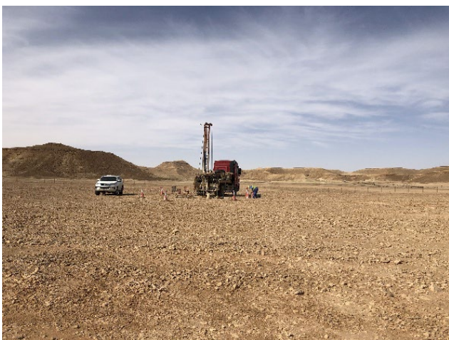
Ground investigation at Wadi Safar near Riyadh, KSA
