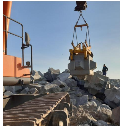
Figure 4 Lifting and placing Cubipods
