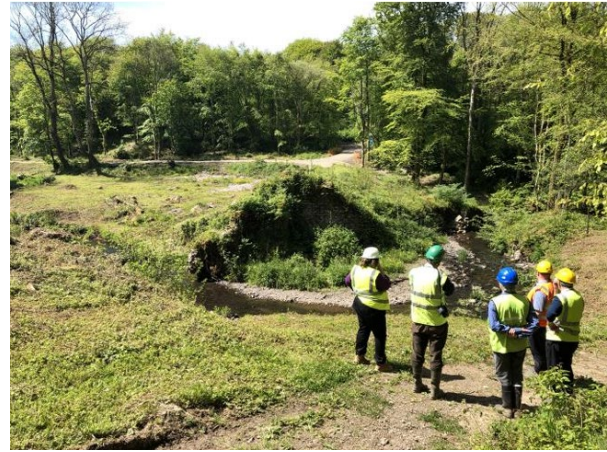
Figure 3 Surveys have revealed structural condition, archaeological remains and environmental assets.
