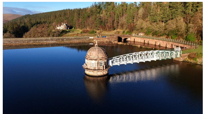
Photo of the Intake Tower at the Talla Reservoir. Credit: David Rankin
