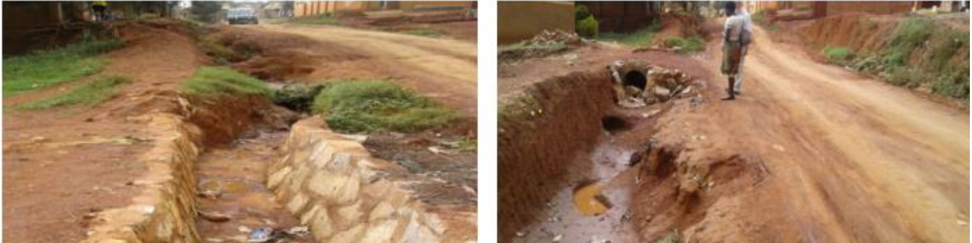
Figure 1 Existing roads and drainage channels
