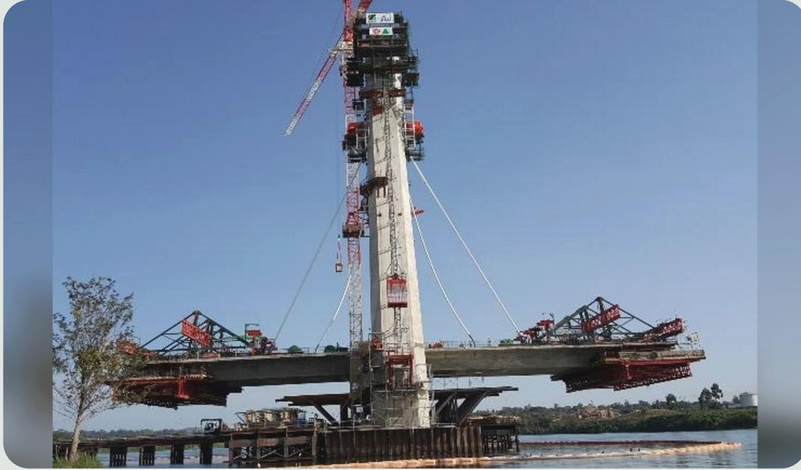
Example of Form travelers advancing the deck from the pylon.
