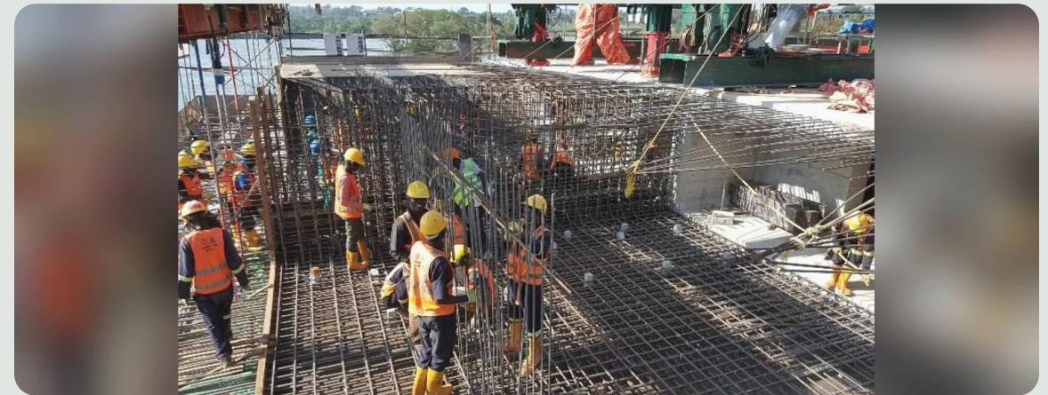
Example of Deck reinforcement and concrete crews at work.
