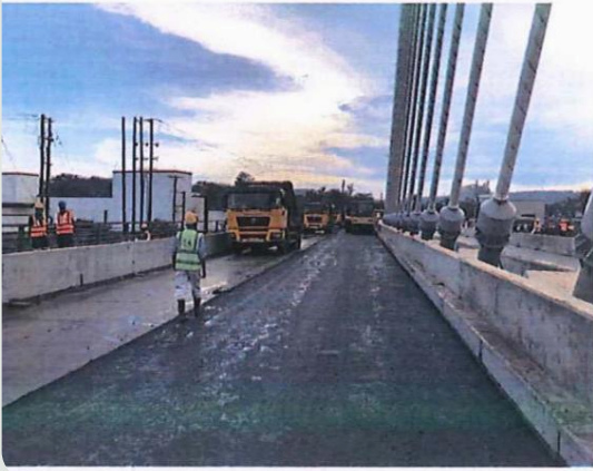
Replacement of asphalt on bridge deck
