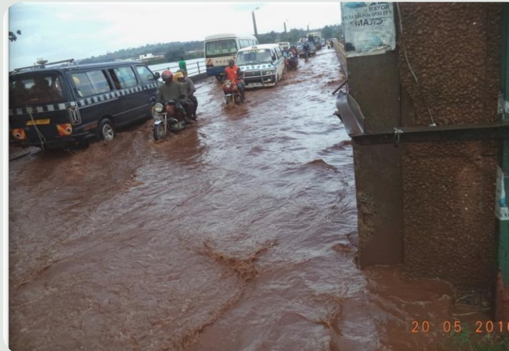
May 2016: flooding and congestion, the daily reality on the old crossing.
