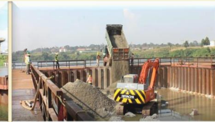
Water displacement in cofferdam
