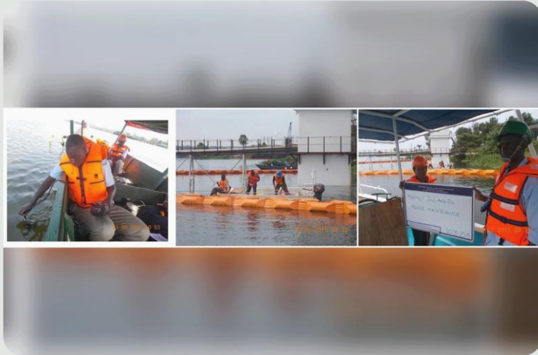
Silt & oil fences around jetties and neighbours' intakes.
