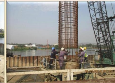
Pile's Reinforcement cage installation
