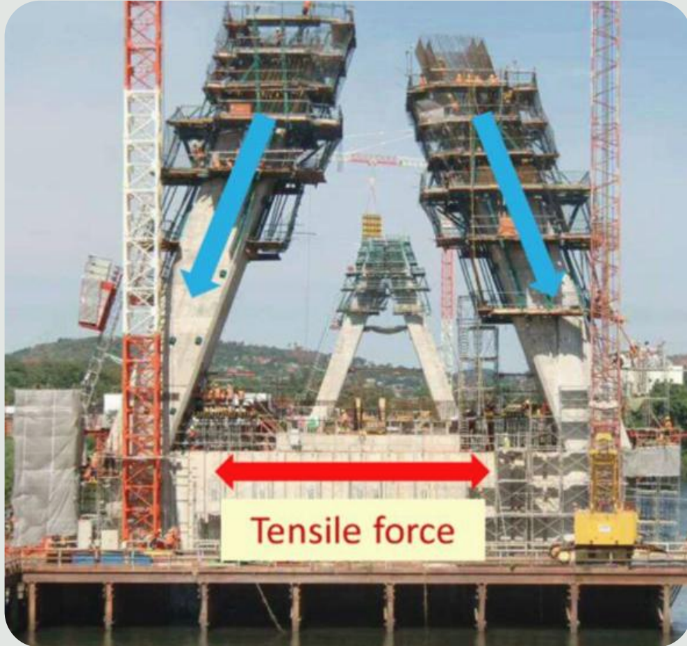
Example of Pylon legs under climbing formwork, tensile forces .
