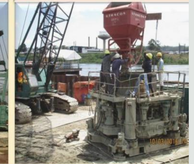
Pile's concrete casting
