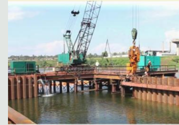
Installation of cofferdam
