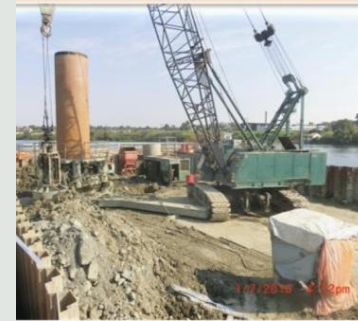
Pile excavation in cofferdam
