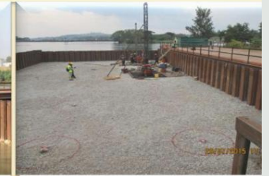
Stabilization in cofferdam
