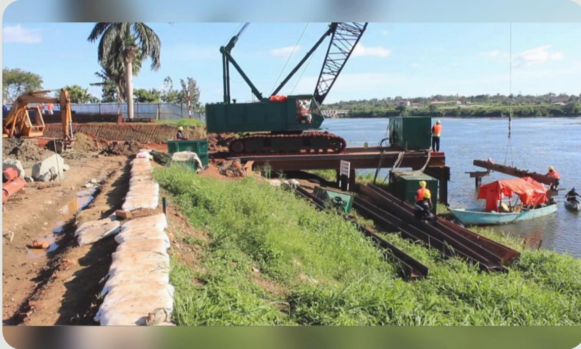
Example of Jetty construction into the water, ahead of cofferdam and piling.
