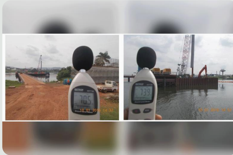
Noise monitoring at the works.
