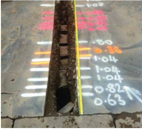
The excavations at Blackwall Reach used a combination of slit trenches and spot excavations to verify critical utility locations using PAS128 survey type A.
