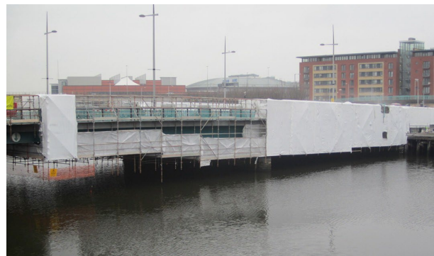
Photo: Encapsulation for repainting works 2012. Credit: DfI
