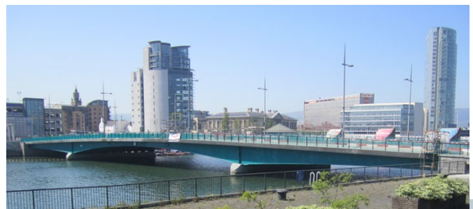
The Queen Elizabeth Bridge spanning the River Lagan, Belfast. Credit: DfI
