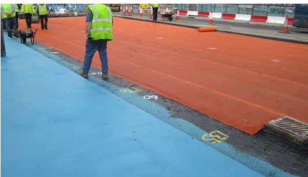
Photo: The Queen Elizabeth Bridge deck joints, anodes and waterproofing. Credit: DfI
