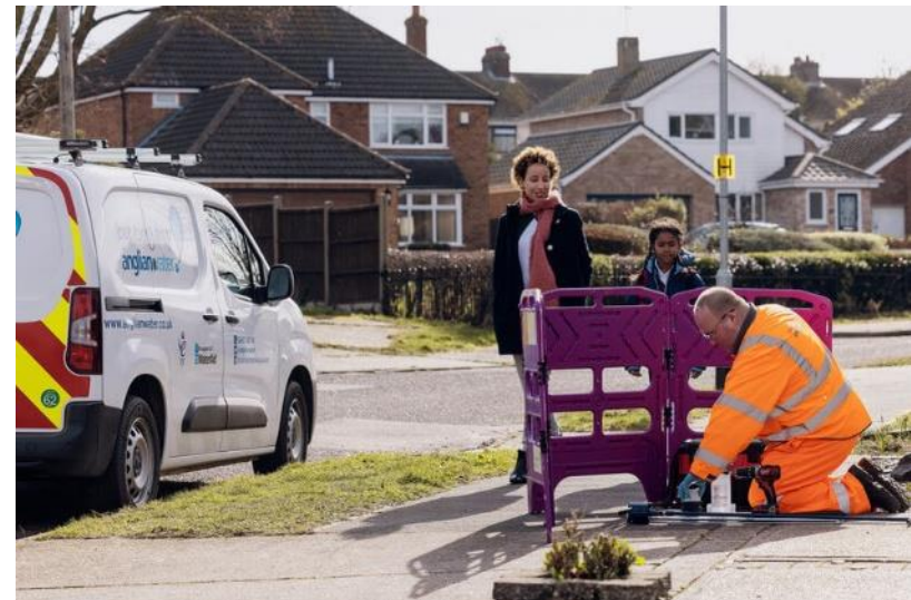
Installation of Smart Water Meters (source Anglian Water)
