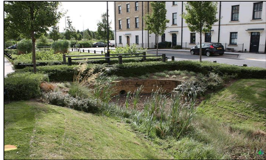
Sustainable Drainage System retrofitted in Mansfield
