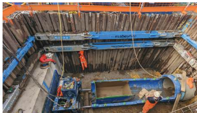
Above: Glynneath Flood Alleviation Scheme
